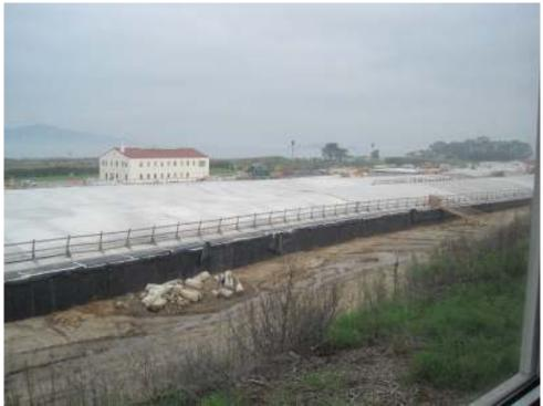
The concrete structures in front of the Observation Post are tunnels on Doyle Drive, which will eventually be covered over with earth and grass and paths so pedestrians will be able to leisurely walk from the main section of the Presidio to Crissy Field without having to dodge cars for dear life.
